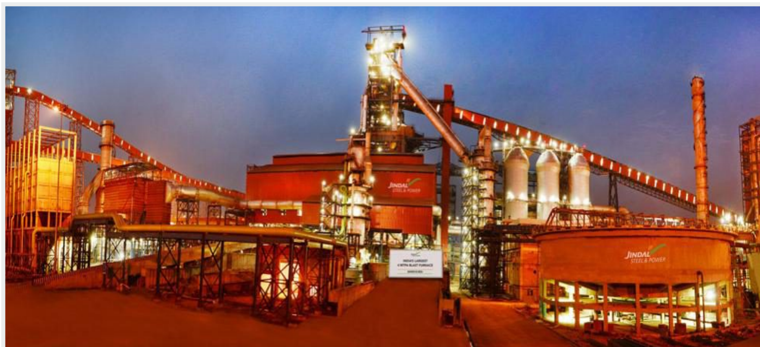
Steel Plant set up by JSPL at Angul
