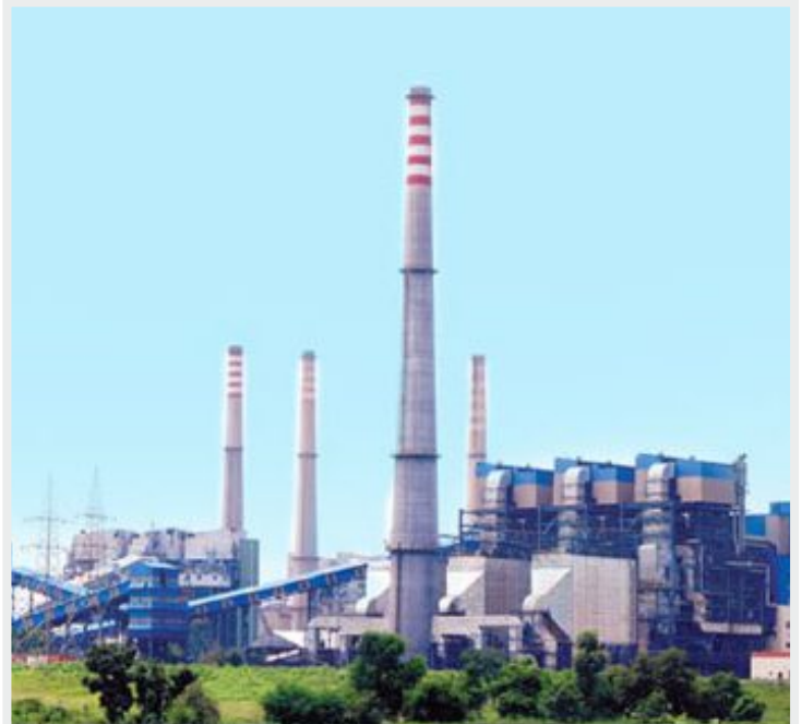
Hindalco Plant at Hirakud, Sambalpur
